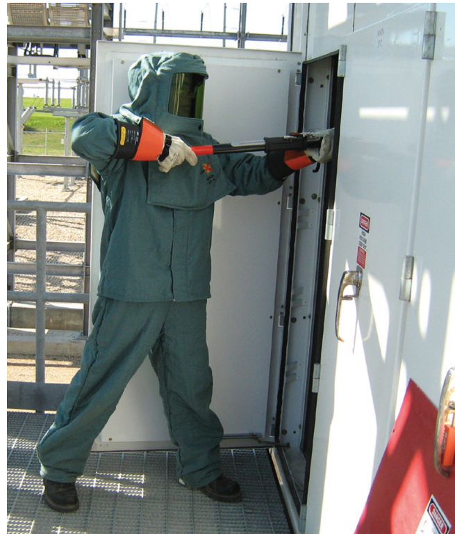
Figure 1-3 An arc flash hazard exists when a person interacts with equipment.
